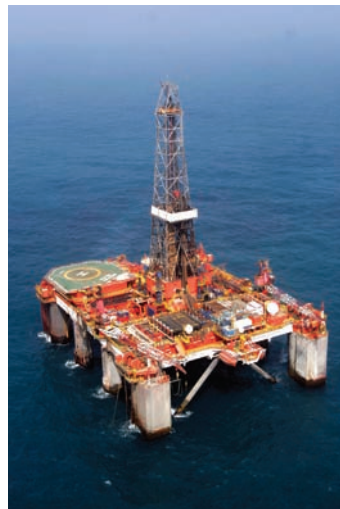
Hurricane Exploration plc
